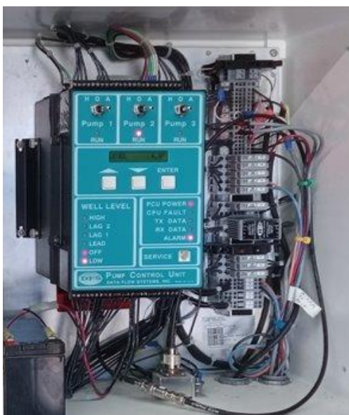
Figure 2: Pompano Beach's initial pump control unit (PCU)
